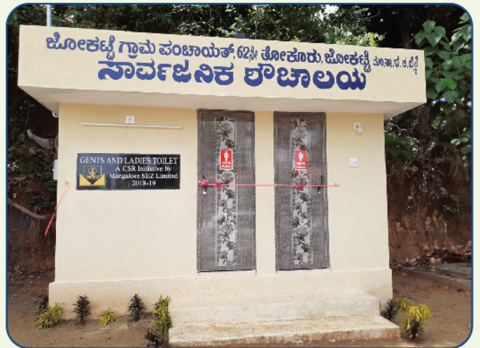
Gents and Ladies toilet block at Jokatte, Mangalore.
