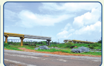
Flyover under Construction
