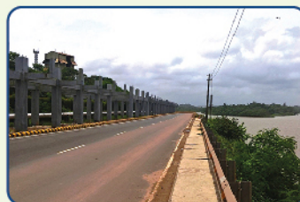
Pipeline cum Road Corridor
