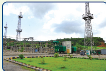
Grid Sub Station
