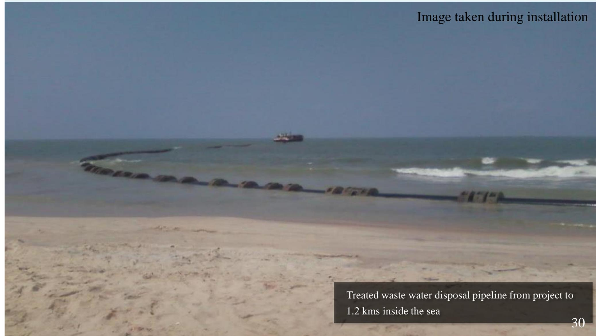
Treated waste water disposal pipeline from project to 1.2 kms inside the sea
